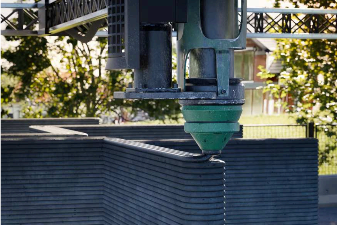
Walls of a house being 3D printed (Shutterstock)
